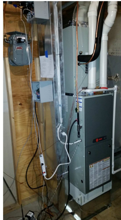
Figure 5 Central ducted air source heat pump system
