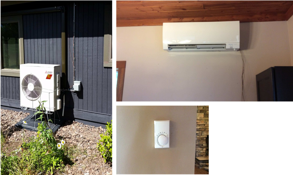
Figure 6 Ductless mini-split heat pump system
