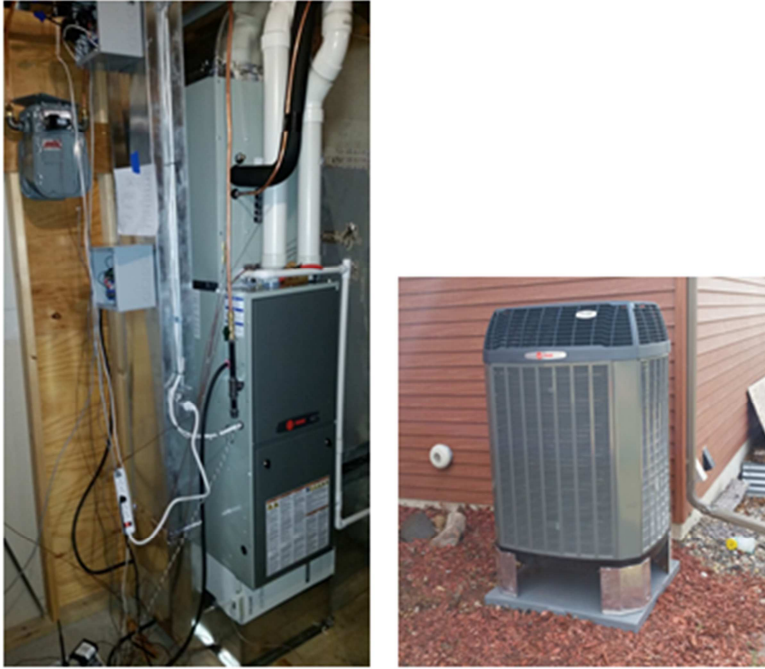
Figure 1. Whole home ducted cold-climate air source heat pump
