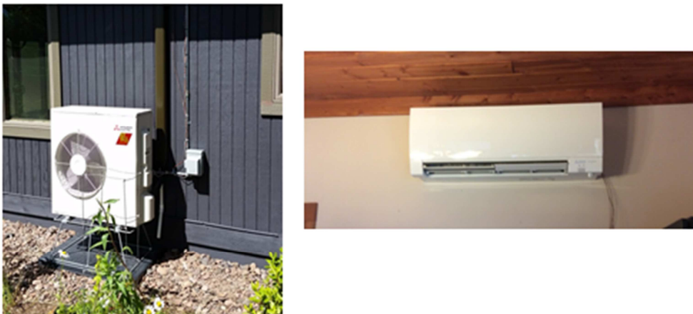
Figure 2. Ductless cold-climate air source heat pump
