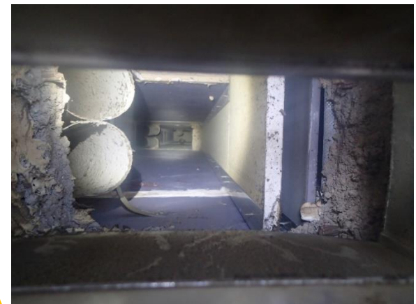
Gypsum shaft , looks discontinuous
