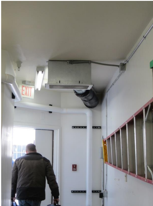
Individual fan in dumpster room
