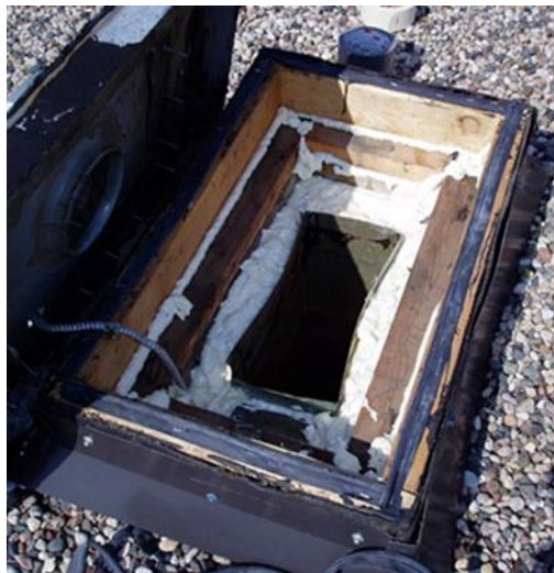
Air seal at curb below fan
