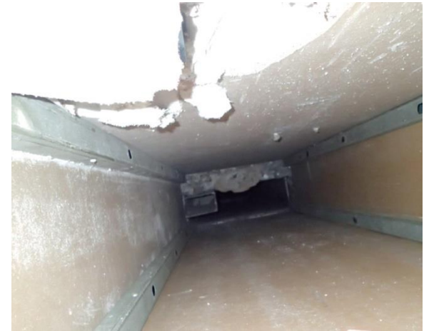
Gypsum shaft , looks discontinuous
