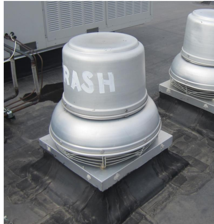
PRV serving trash rooms (on each floor) and dumpster room
