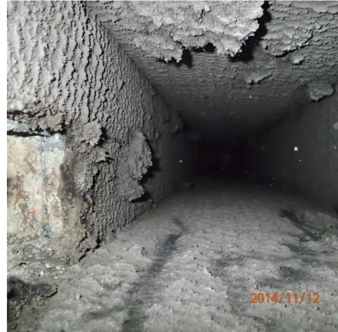
Lined duct in roof cavity
