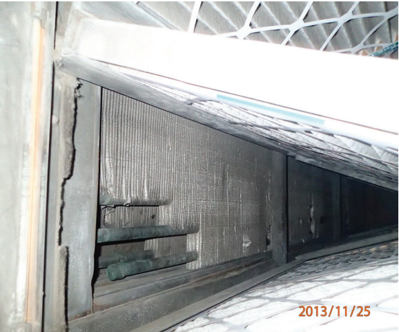
Figure 6: Dirty heat exchange coil restricted airflow. Air was bypassing the filters (right side) because of a broken hinge on the filter access door and dust was accumulating in the heating coil in the air handler, affecting heating efficiency and restricting airflow.
