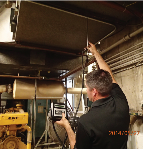
Figure 8: Test and balance contractor measuring airflow before and after fan turn down.
