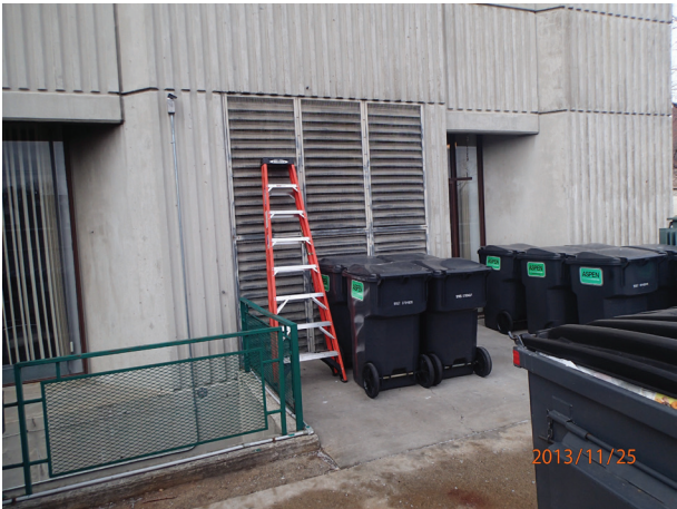
Figure 2: Air intake for corridor air handling unit
