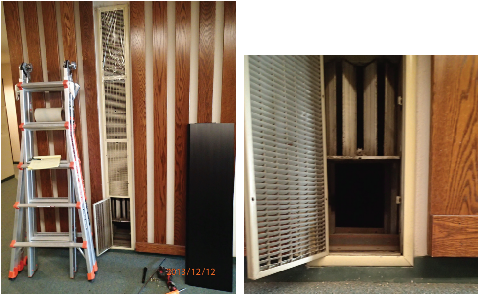
Figure 3: Corridor registers. Left: A single 8”x80” register supplies make up supply air to each floor’s corridor. Right: The balancing damper behind the register grille provides airflow adjustment.
