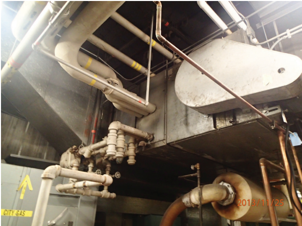
Figure 1: Corridor supply air handling unit
