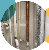
Drain water heat recovery coil
