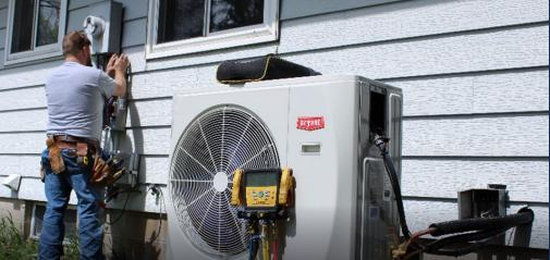
Air source heat pump being installed and paired with a ducted gas furnace at a Twin Cities Habitat for Humanity house in Rosemount, Minnesota
