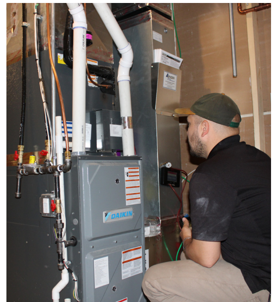
From left, the TCHFH new home in Minneapolis during final testing and a CEE rater setting up to test the external static pressure of the HVAC ducting system.
