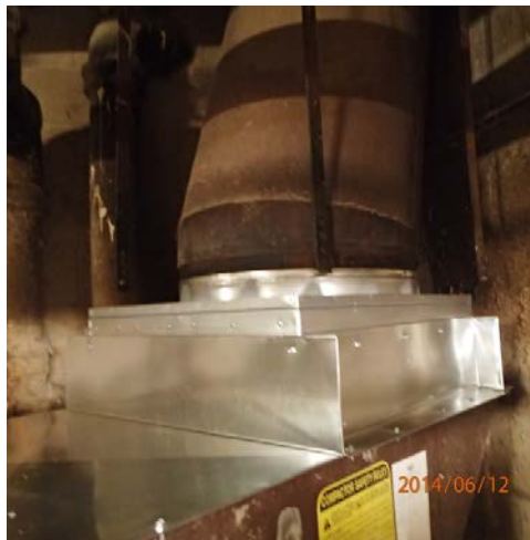
Chute sealed to the compactor with sheet metal
