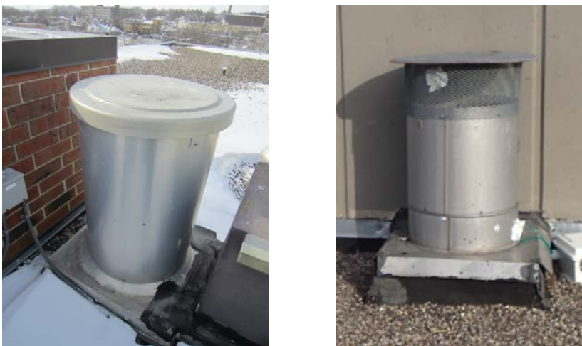
Figure 14. Trash chute rooftop terminations
