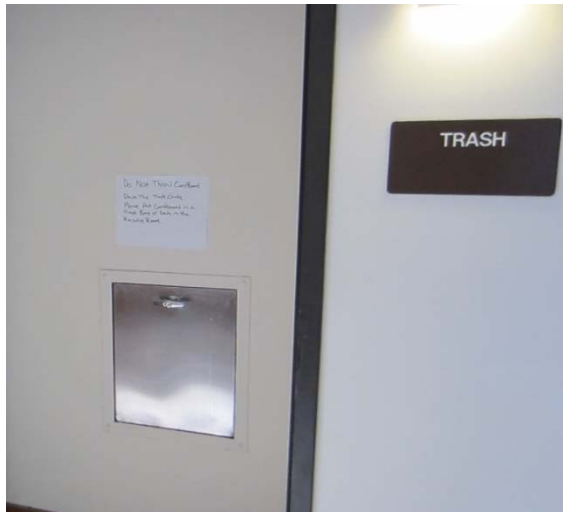
Figure 16. Trash disposal access from hallway
