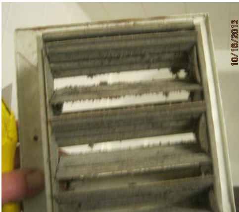
Figure 2a. Balancing louver integrated with inlet grille
