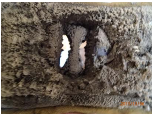
Figure 3a. A very dirty Constant Air Regulating (CAR) automatic balancing orifice
