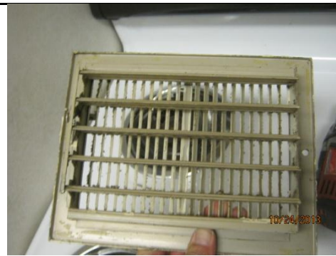
Fig 4. Adjustable dampers: remove, fix open, or use fixed grille
