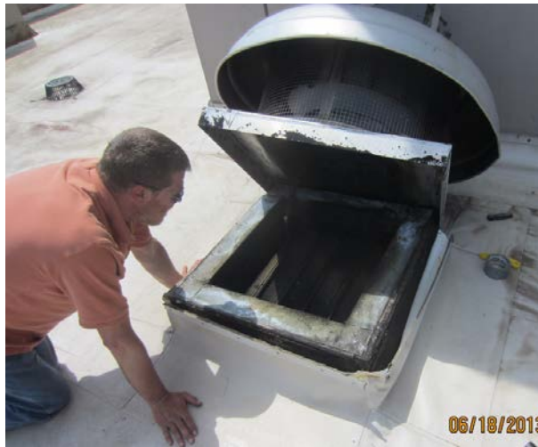
Figure 7. Duct leakage at roof curb below PRV fan
