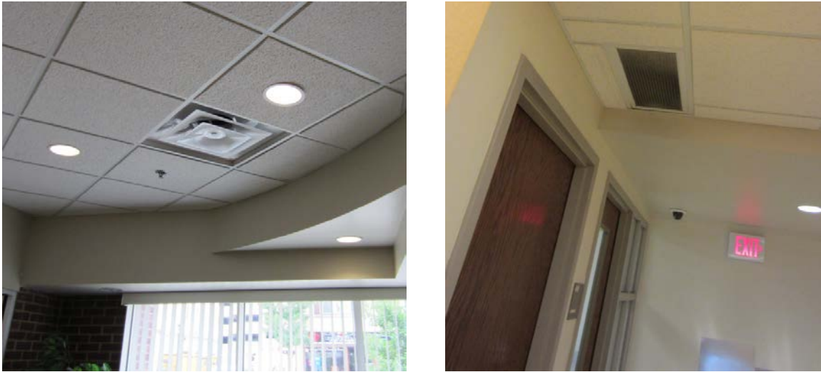
Figure 12. Register grilles
