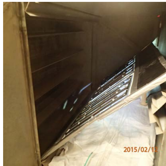
Figure 25. TrueFlow meters installed into an outdoor air intake duct
