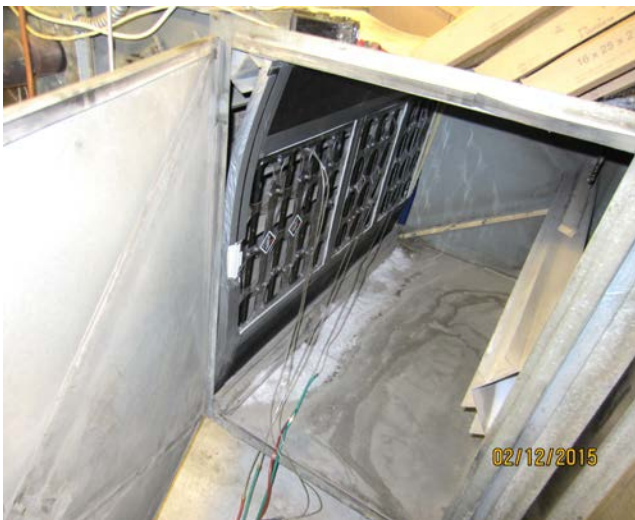
Figure 25. TrueFlow meters installed into an outdoor air intake duct
