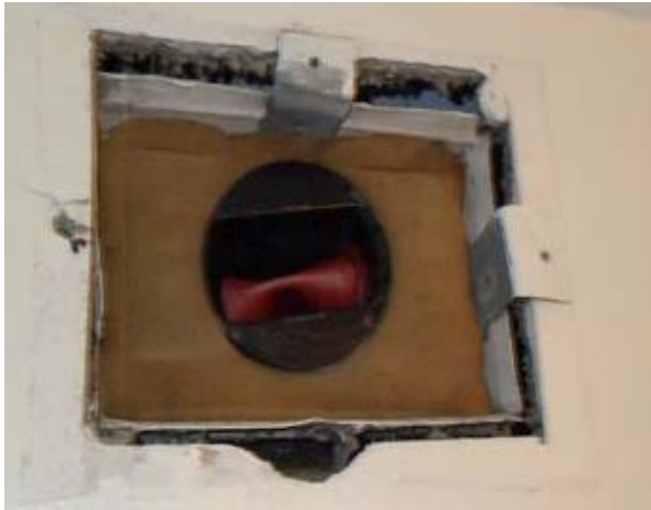
Figure 8. Duct leakage around exhaust inlet
