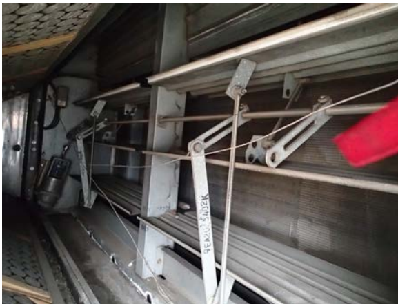
Figure 11a. Air damper actuator failed in open position
