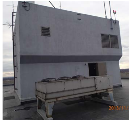
Figure 5b. Exhaust grille on penthouse wall.
