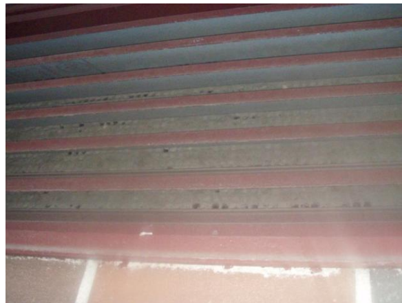
Figure 11b. Close-up view of clogged air intake bird screen
