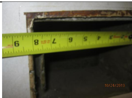
Fig. 6 Orifice plate with 2.45 inch reducing washer, 2 bedroom
