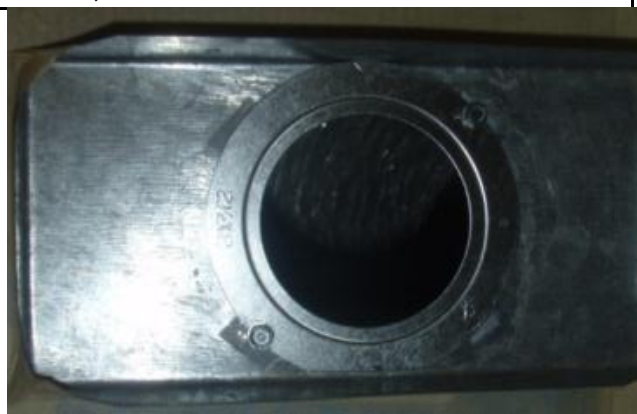
Fig. 6 Orifice plate with 2.45 inch reducing washer, 2 bedroom
