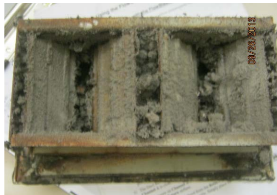
Figure 3b. A dirty balancing louver
