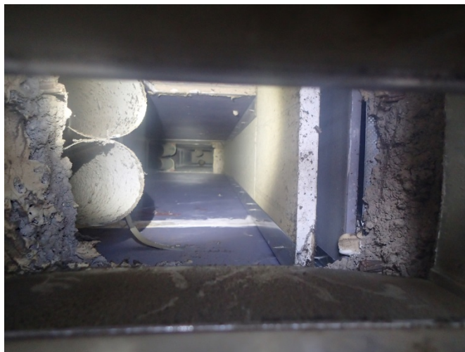
Figure 7. Duct leakage at roof curb below PRV fan
