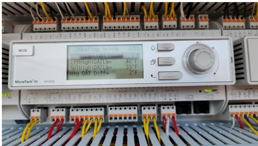
This control sequence explains why the system occasionally used gas at moderate ambient temperatures, but it does not explain why the system was able to enter heat pump heat + gas heat or defrost + gas heat modes.
