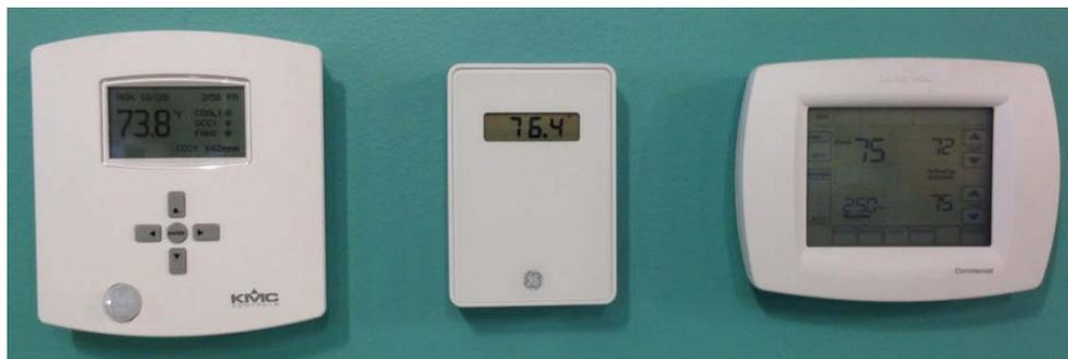
CEE consulted again with the manufacturer about this observed space temperature error. In response, the manufacturer issued a calibration procedure that was required if there appeared to be an issue with the space temperature reading. This calibration procedure can be found on the internet under CO2 FlexStat Temperature Offset (document SB0412A).
