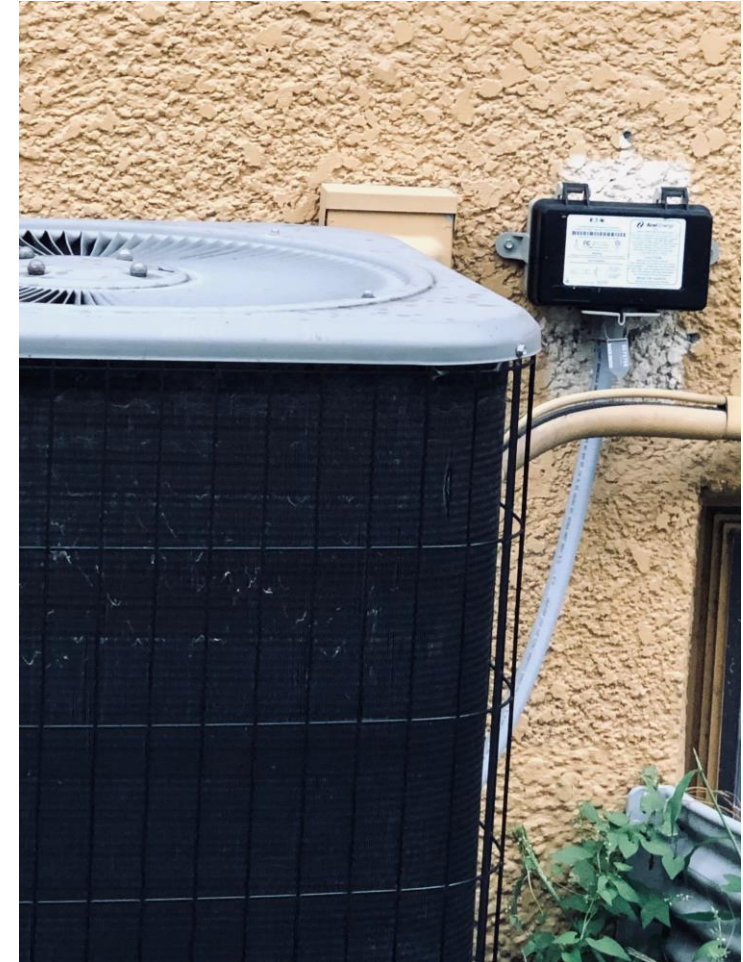
Presenter's Direct Load Control Switch on AC Unit
