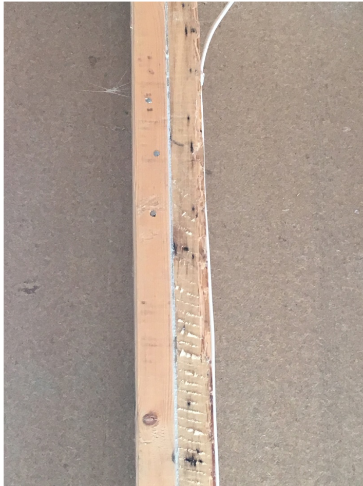
Figure 74. Seal gap between framing
