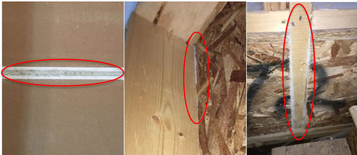
Figure 35. Example aerosol seals: gap between drywall sheets (left), gap between framing and sheathing (middle), and rim joist gaps (right)
