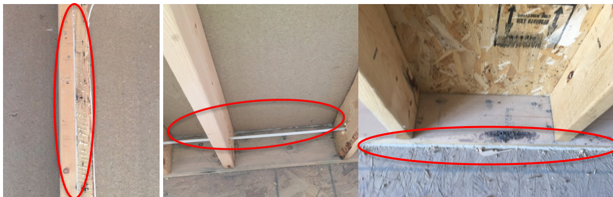
Figure 38. Example aerosol seals: between framing (left); between sill plate/sheathing; between sill plate/subfloor
