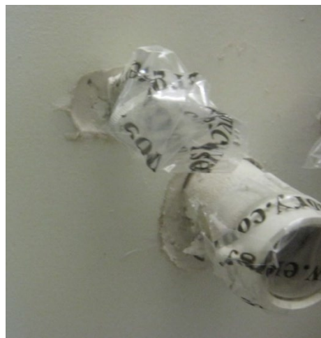
Figure 68. Temporary cover over open plumbing pipes
