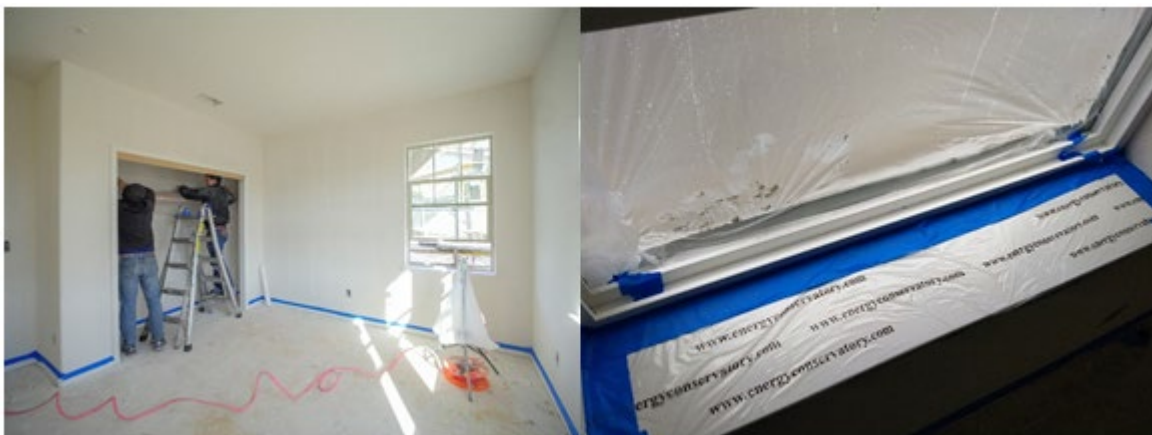
Figure 24. Additional preparation required in Houses #9, #10, and #11 to protect installed trim, including baseboards and shelves (left) and windowsills (right)
