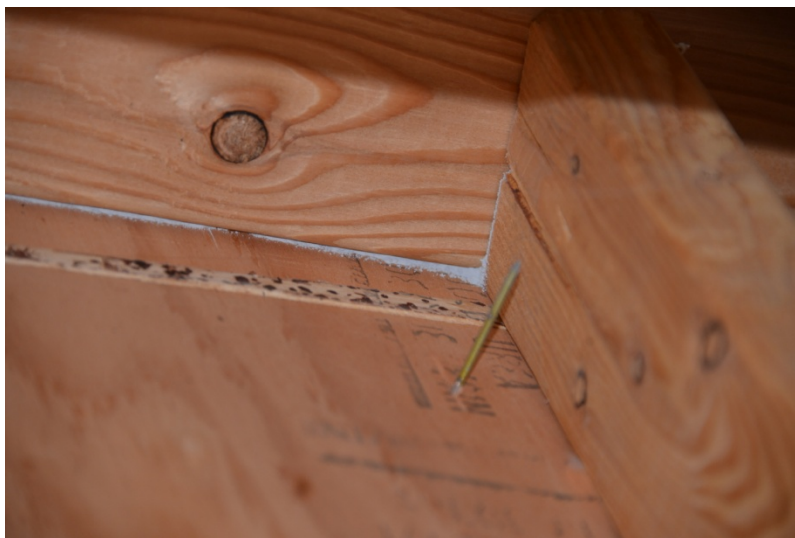
Figure 75. Seal between sheathing and framing
