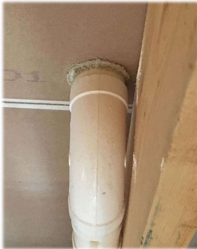
Figure 73. Seal between plumbing penetration and drywall
