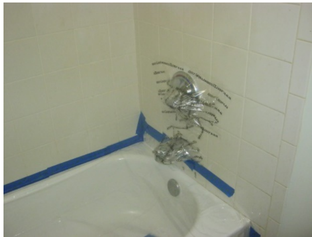
Figure 69. Temporary cover over tub and plumbing fixture
