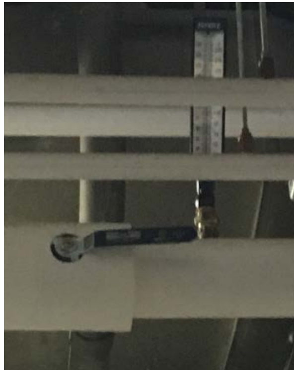
Figure 24. In-line temperature sensor that was replaced for the controller flow sensor
