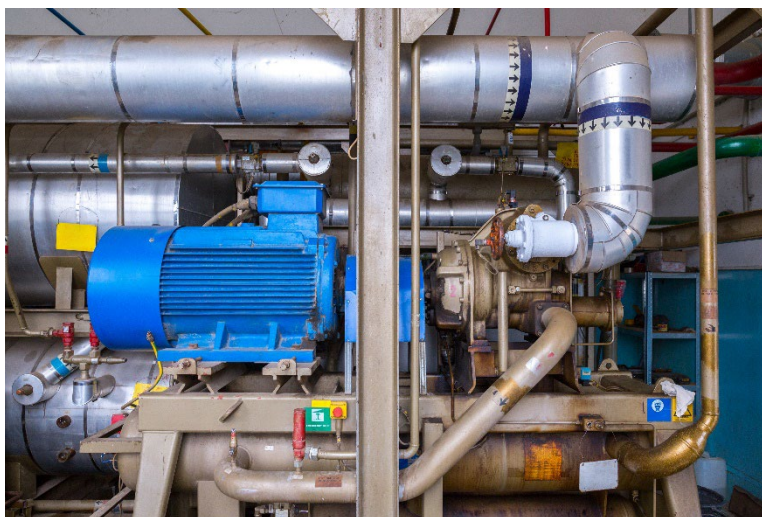
Figure 1: Ammonia Screw Compressor
