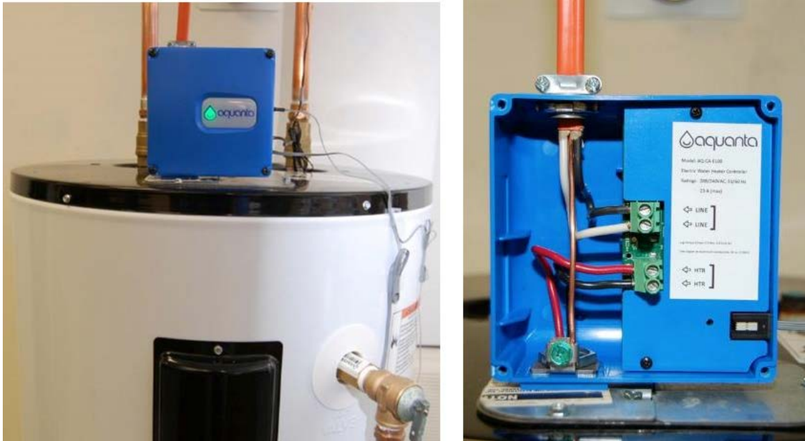
Figure 4. Aquanta Unit Installed on an Electric Storage Water Heater
