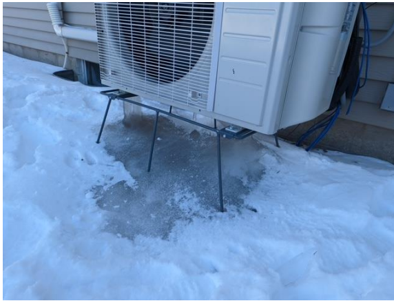
Figure 18. Ice buildup under an ASHP outdoor unit
