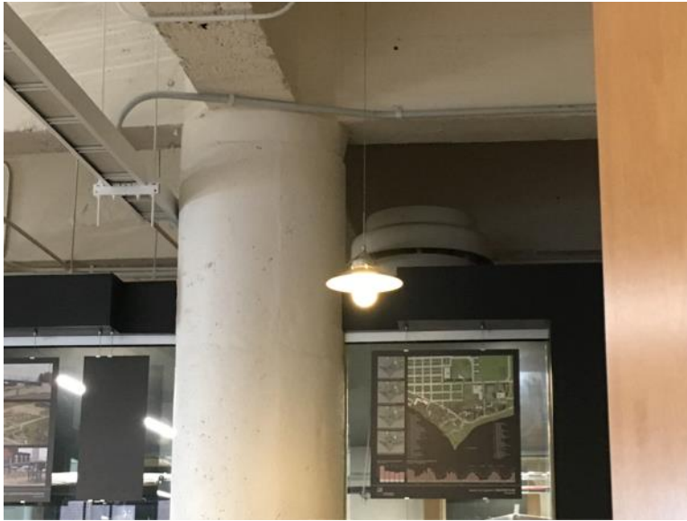
Figure 31. Transfer Grille into Server Room at Site 2
