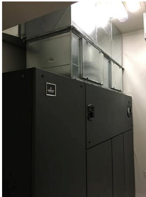
Figure 10. Computer Room Air-Conditioning Unit (CRAC)
