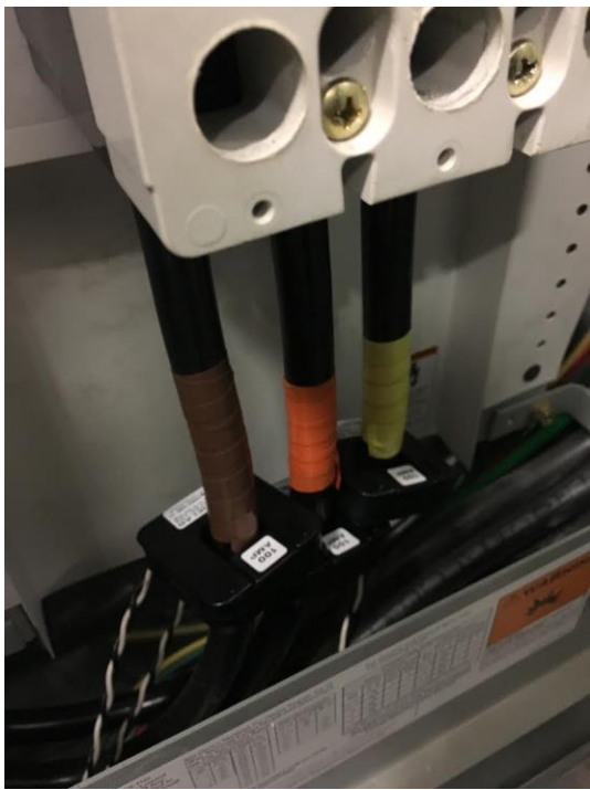
Figure 15. Panel-Installed CT Clamps
