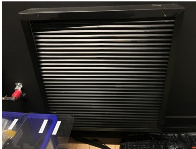
Figure 31. Transfer Grille into Server Room at Site 2
