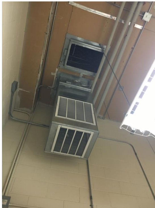
Figure 33. RTU Supply and Return at Site 7
