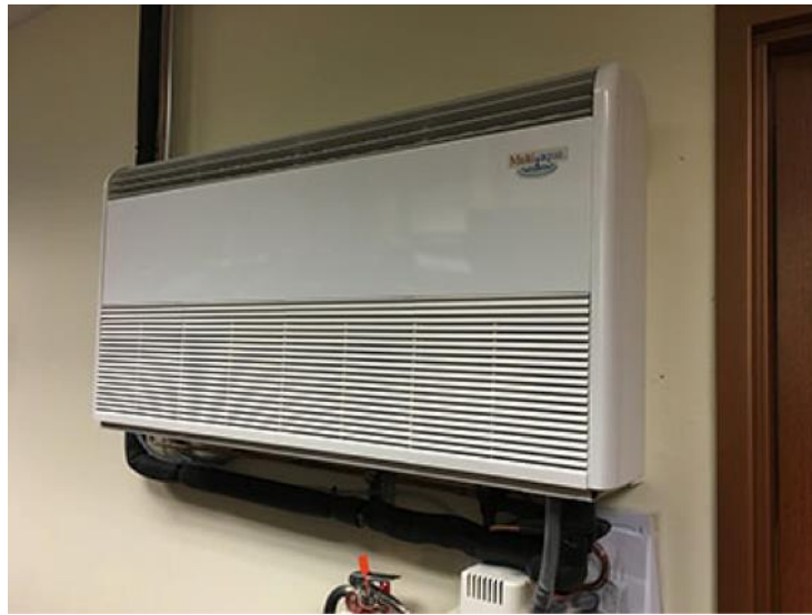
Figure 10. Computer Room Air-Conditioning Unit (CRAC)
