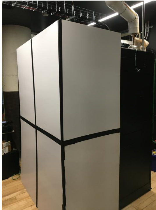
Figure 60. Filler Panels Installed in Site 2 Server Racks
