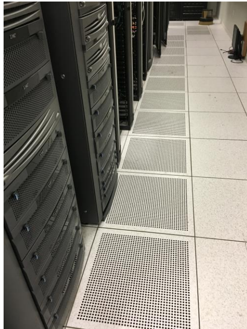
Figure 27. Under Floor Cold Air Supplies at Site 1
