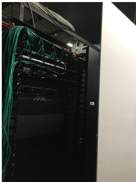
Figure 60. Filler Panels Installed in Site 2 Server Racks
