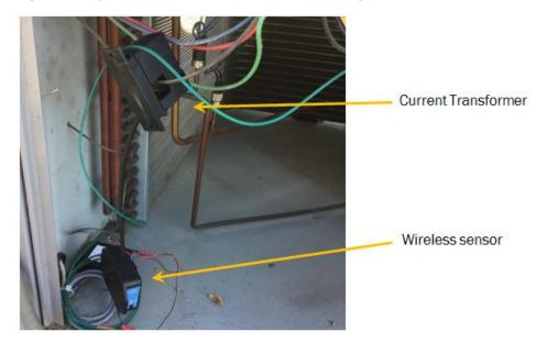
Figure 32: Typical electric consumption monitoring installation
