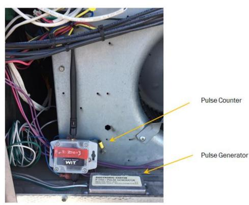
Figure 31: Typical gas consumption configuration
