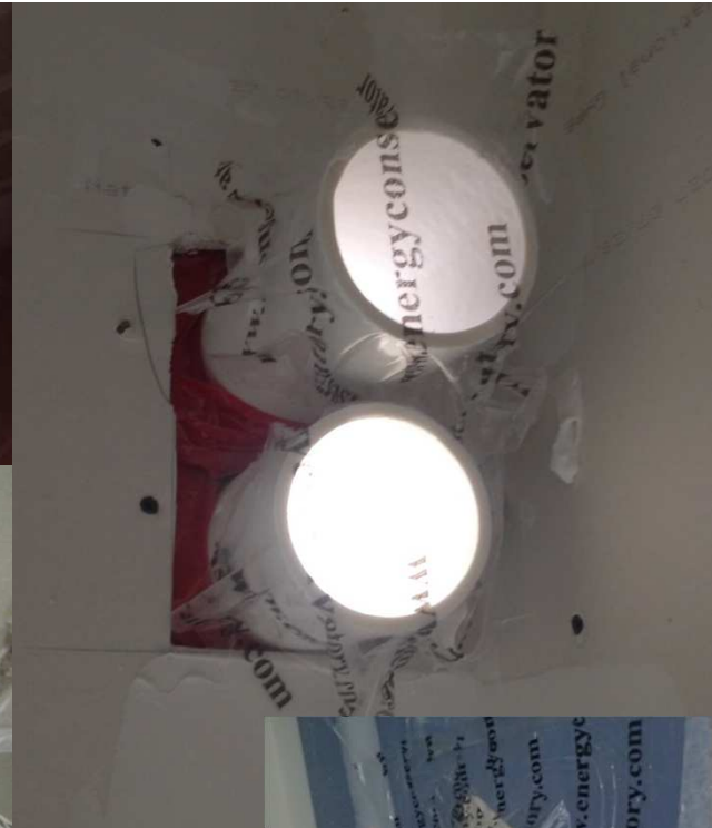
Combustion vents
