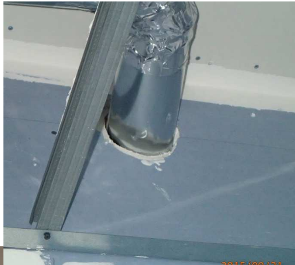
Duct penetration
