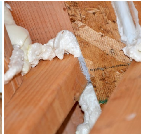
Aerosol sealing installation on a single-family home including examples of seals formed. Photos from UC Davis WCEC
