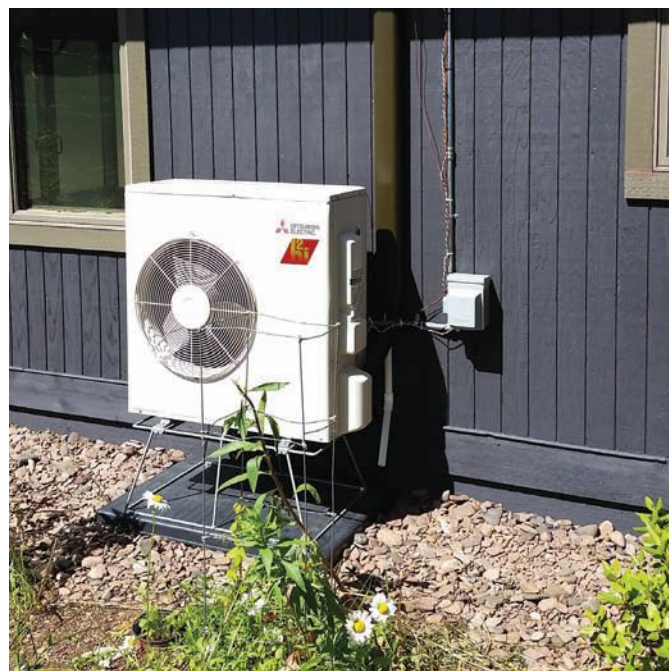
Ductless cold-climate air source heat pumps (ccASHP) inside and outside units. The wires hanging down from the indoor unit are part of the testing equipment.
