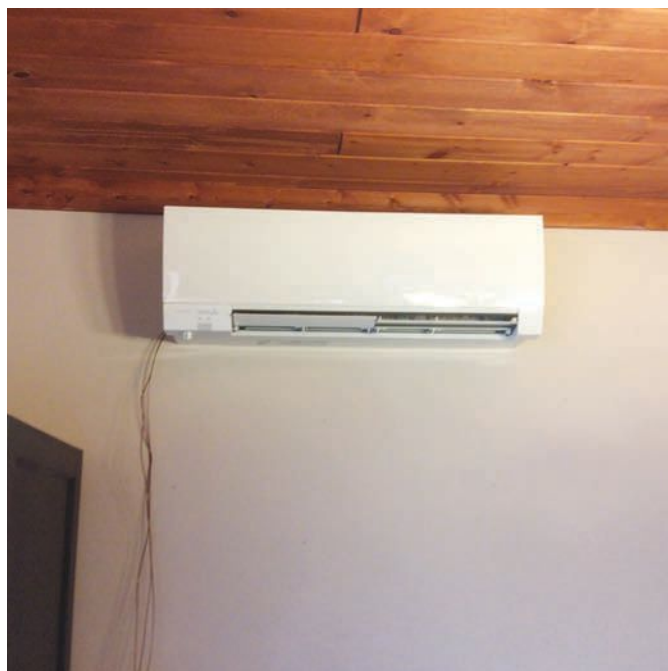
Ductless cold-climate air source heat pumps (ccASHP) inside and outside units. The wires hanging down from the indoor unit are part of the testing equipment.
