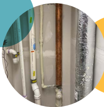
Drain water heat recovery coil
