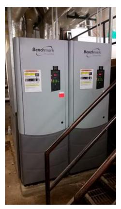
Figure 35. Example of a condensing boiler in a commercial application.
