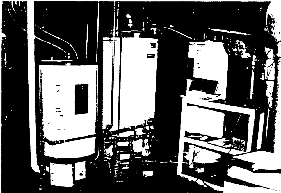
High Efficiency Heater, Existing Heater, Storage Tank (L to R) at Site 2
