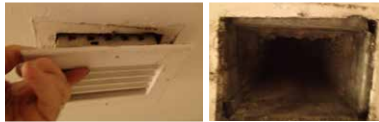
Figure 9: Before installation. Air leakage often found around the duct where it meets the sealing is important to seal.
