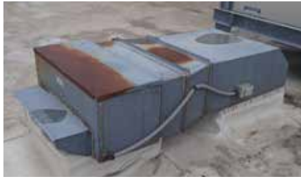
Figure 3.1 & 3.2: Exhaust PRVs on rooftop. Large PRVs on the roof provide exhaust flows ranging from 850 to 1,850 cfm. One PRV had an unusual termination cap that required modifications to our flow capture boxes.
