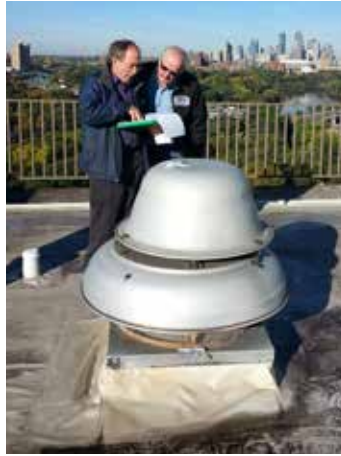
Figure 3.1 & 3.2: Exhaust PRVs on rooftop. Large PRVs on the roof provide exhaust flows ranging from 850 to 1,850 cfm. One PRV had an unusual termination cap that required modifications to our flow capture boxes.
