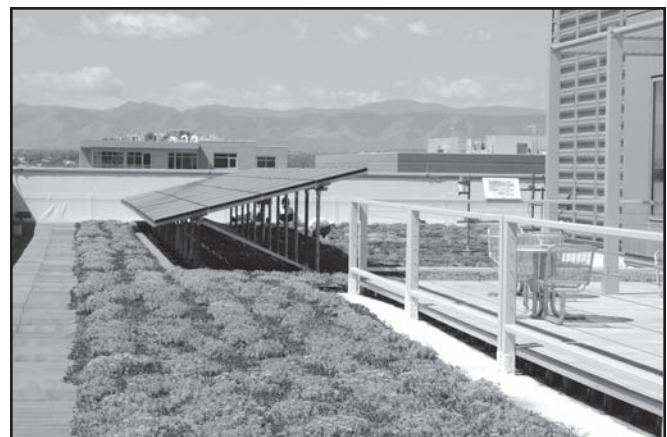
Figure 12. Part of the photovoltaic structure at the Region 8 Environmental Protection Agency Headquarter's green roof. Photo courtesy Thomas J. Slabe.
