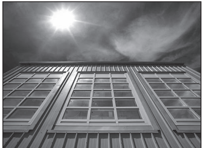
Figure 8. West facing windows absorb heat through the sun. The principle behind the proposed technology uses nanocrystals synthesized chemically to absorb near infrared light and inhibit solar heat gain, while staying transparent so that the coating does not interfere with visible light transmittance. Photo courtesy Delia Milliron and Lawrence Berkeley National Laboratory.
