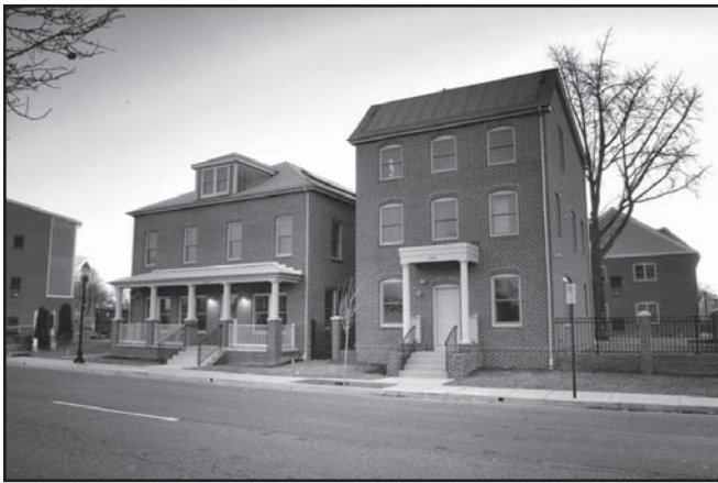
Figure 13. North Pointe Community in Frederick, Maryland. Photo courtesy NEXUS EnergyHomes, Inc.
