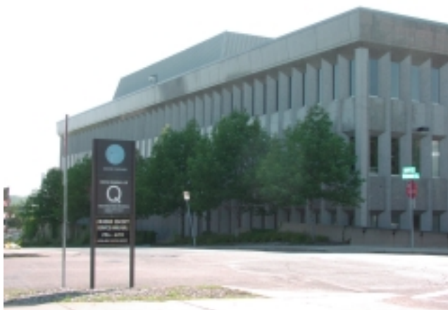
Figure 1. Front view of office building
