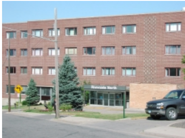
Figure 1: Front view of extended-care mental health facility.
